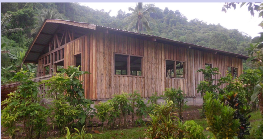
Above: New Dining Hall nearly ready for children
